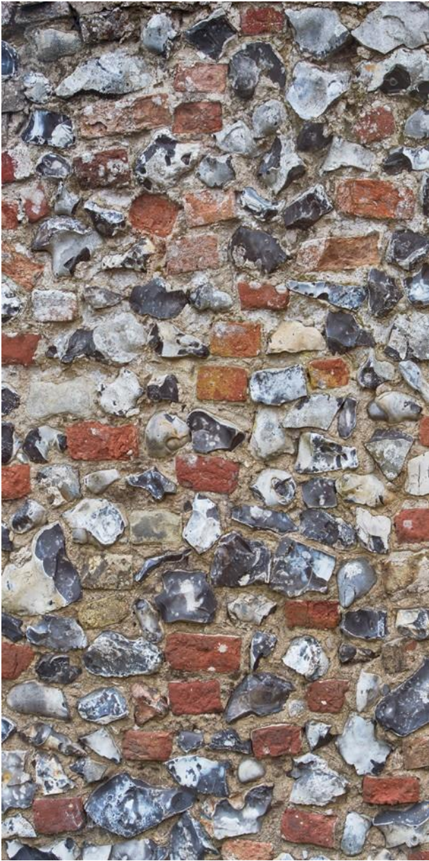
V14T55 Flint and Brick Wall 1
